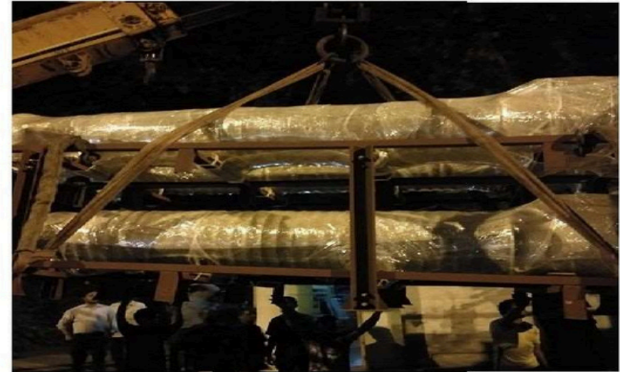
420 KV CV (Chabra Terminal Power Plant)
